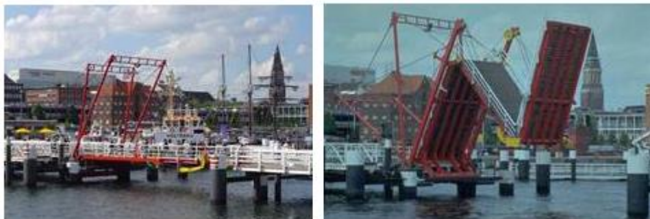
Figure 4-6 Hörn Bridge at Kiel, Germany
